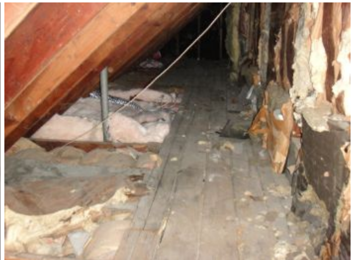
Attic Insulation Condition
