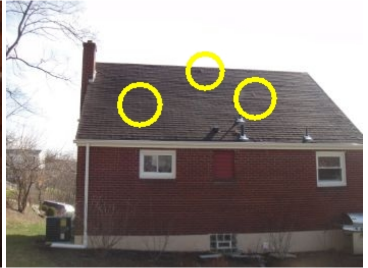
Roof Roof Condition
